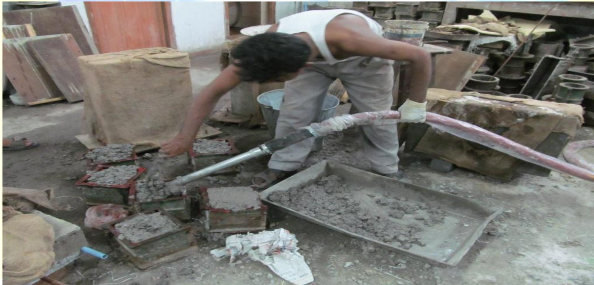
Figure 4 Geopolymer concrete casting
