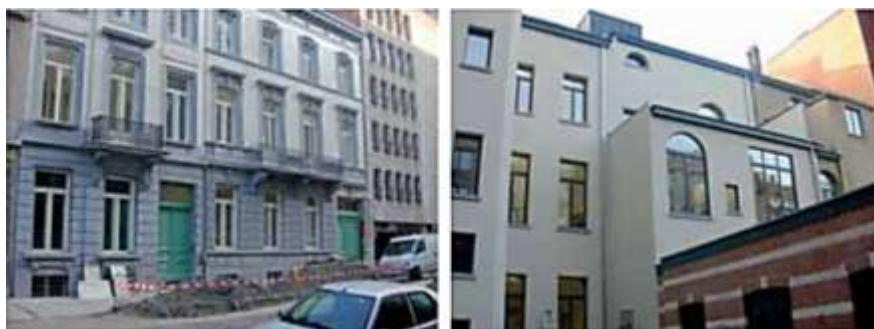
Figure 1: Before and after shots of the renewable energy home in Brussels
