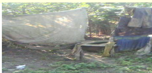
Photo 8: Poor Sanitation System of tea workers
