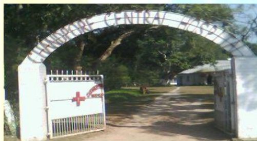
Photo 3: Central Hospital at Tea Garden
